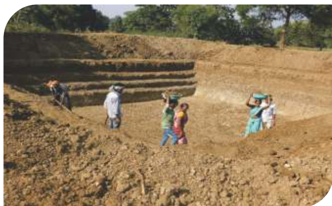
Farm Pond Excavation at Kalahandi Unit
